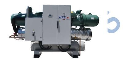
Unit capacities are listed in the performance data section. Intentionally over-sizing a unit to assure adequate capacity is not recommended. Erratic system operation and excessive compressor cycling are often a direct result of an oversized chiller. In addition, an oversized unit is usually more expensive to purchase, install, and operate.
